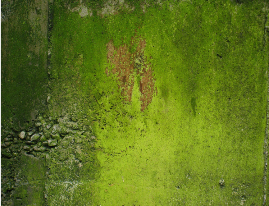
ABOVE: Made by Taiwan Series/Roadside: North-Facing Retaining Wall #1, 2009. Karen McCoy
